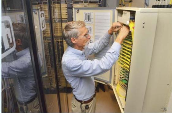
The fiber distribution system uses only part of the conduit and needs only a 2- by 3-foot cable box. “The frames go away, and the walls are bare and the tray empties,” said Sandia Senior Engineer Steve Gossage
